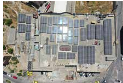
■ Solar panels on the roof of the bus station.
